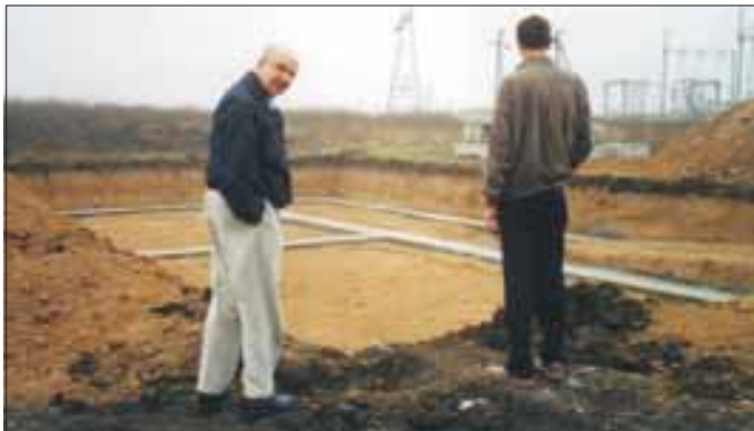
Dr. Threinen inspects the foundation work for the seminary in Ukraine
