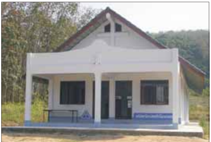
Kok Kloi church needs a portable gasoline generator.
